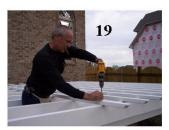
Set the clutch on the drill to insure that the screw head does not dimple the top surface of the purlin. Continue across the top of the rafters until all purlins have been in-
