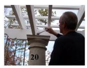
Using a 15/16" deep well ratchet or opened end wrench tighten the nut on top of each columns until very tight.
