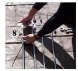
Attach a connector nut to the threaded rods and then attach the short six inch stainless steel threaded section to the top of the connector nut.
