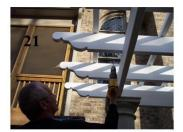
Using a 1/8" drill bit drill a hole in the bottom near the end of each header, rafter, and purlin. This will insure that moisture will vent should any collect.
