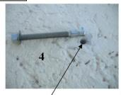
Use the hammer to Install the stainless steel anchor in the prepared hole
