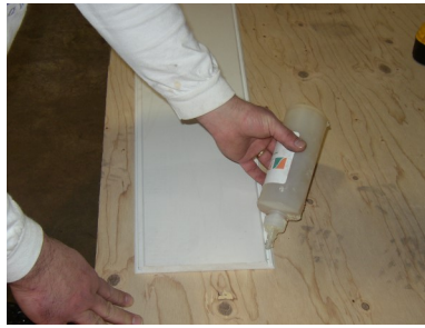
11) Apply adhesive to final panel.
