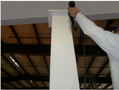
13) Apply glue to final 1/4 cap piece and biscuits and slide into place. Pin nail cap moldings to top of column.*
