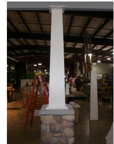
18) Clean surface of column with cleaner recommended by the paint manufacturer. Paint with 2 coats of acrylic latex paint.
