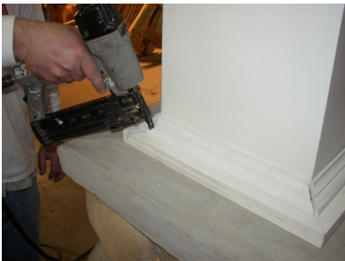
16) Center trim moldings around shaft. Apply adhesive to base trim moldings and pin-nail into base platform. (Do not attach to shaft.) There should be about a 1/16" gap around shaft.
