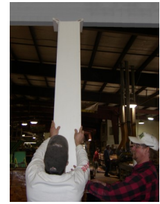
12) Assemble final panel to column using miter joint. Nail panel to secure in place.
