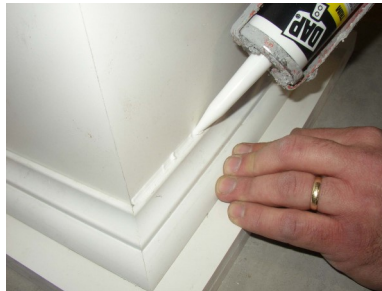
17) Caulk using latex caulking compound to fill any gaps and nail or screw holes.
