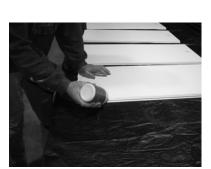
3) Apply polyurethane glue to both edges of ONE PANEL only.
