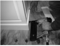
8) Apply glue to backs and mitered edges of base moldings, then assemble to bottom of platform (same as no-taper column bases).
